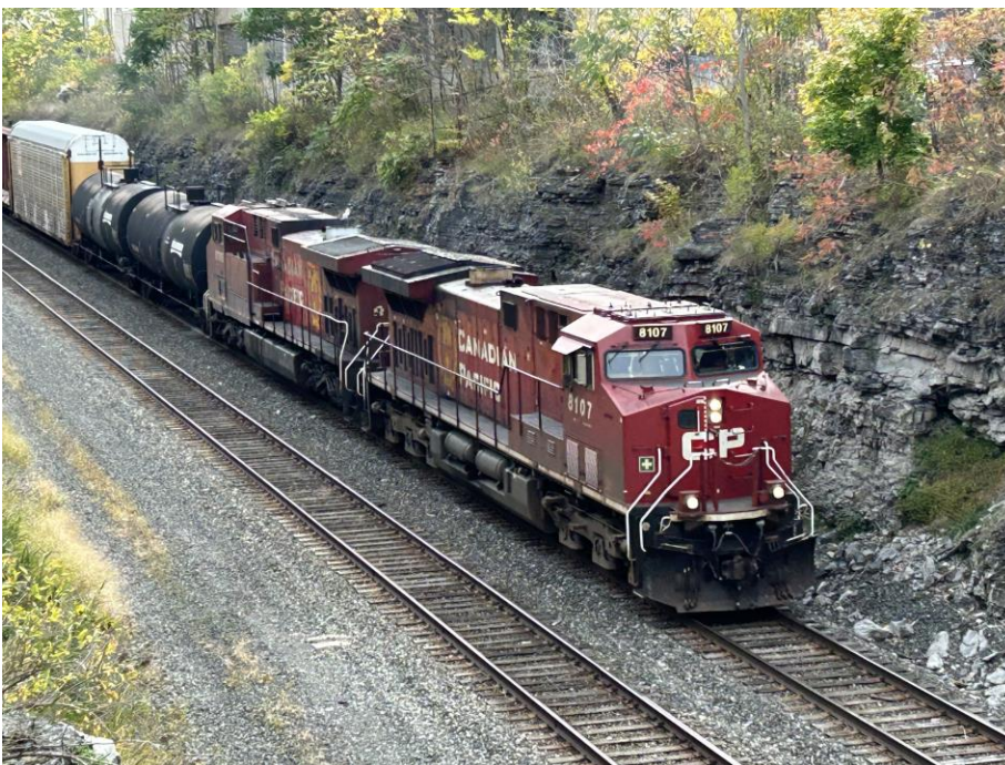
CP Rail's freight transfer to Fort Erie is on the Belt Line in Buffalo, NY near the Dewey Avenue overpass. Much of the Belt Line is below grade in this part of the city, work that was undertaken over 100 years ago. Notice that there was at one time a third track in this area on account of the once dense amount of industry along the route. October 19, 2023. Larry Gustina photo.
