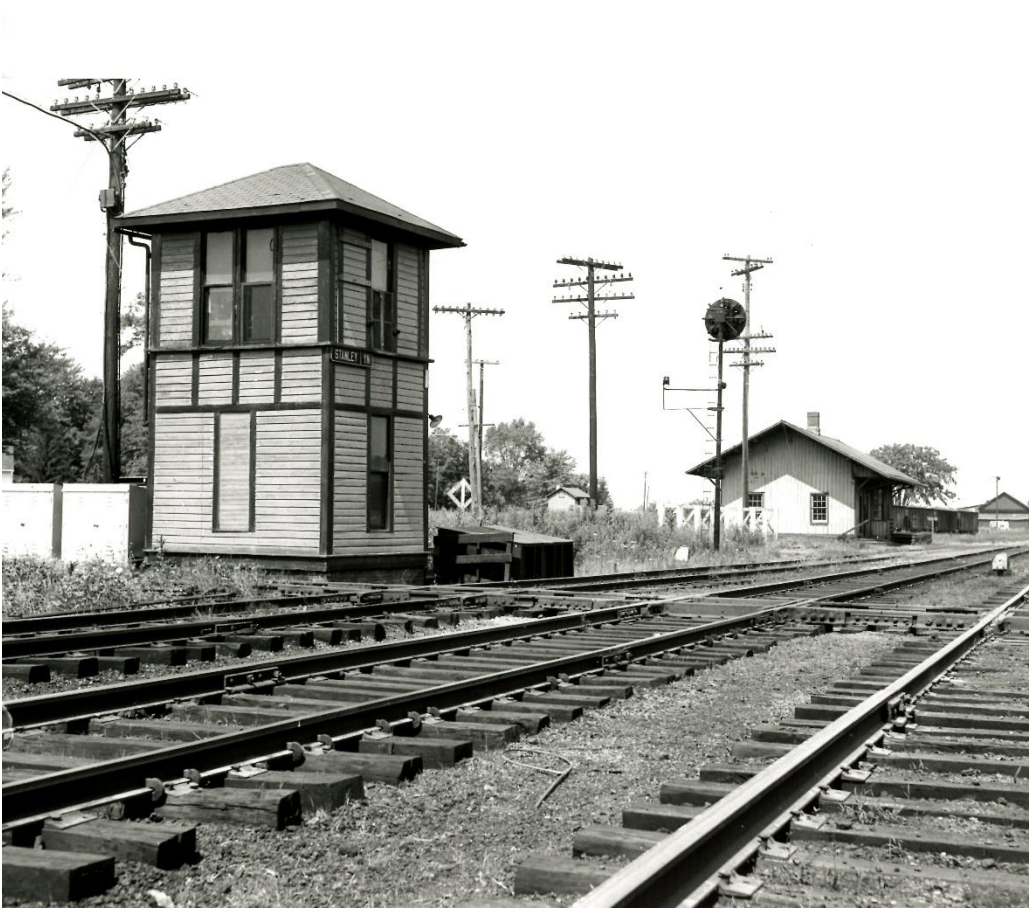
Stanley Tower, about 1952. Here we are looking along the Pennsy's branch and their station is in the distance. Note the PRR position light signal which guards the diamond.
